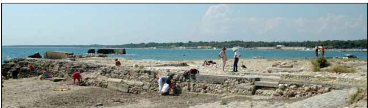
Below: The pier undergoing cleaning and recording during the study of relationships between the port and the Roman and medieval town at Lecce
