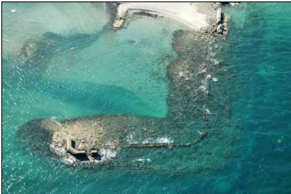
Left: The remains of the Roman pier at San Cataldo, showing how the ancient structure was re-used when the modern pier was built on top of it in 1901
